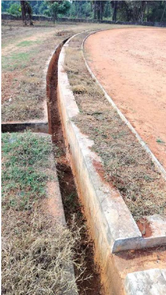
RAIN WATER DRAINAGE SYSTEM AT 400 MT. RUNNING TRACK
