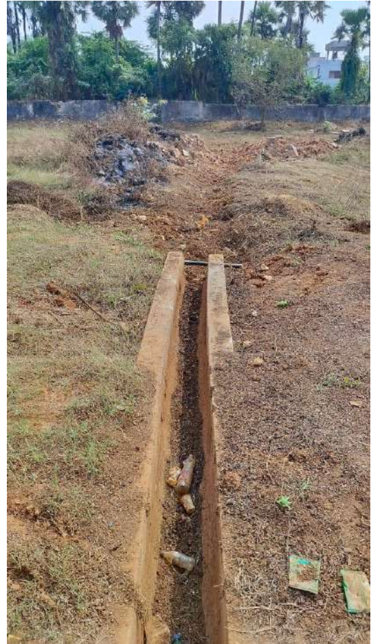
RAIN WATER DRAINAGE SYSTEM AT 400 MT. RUNNING TRACK
