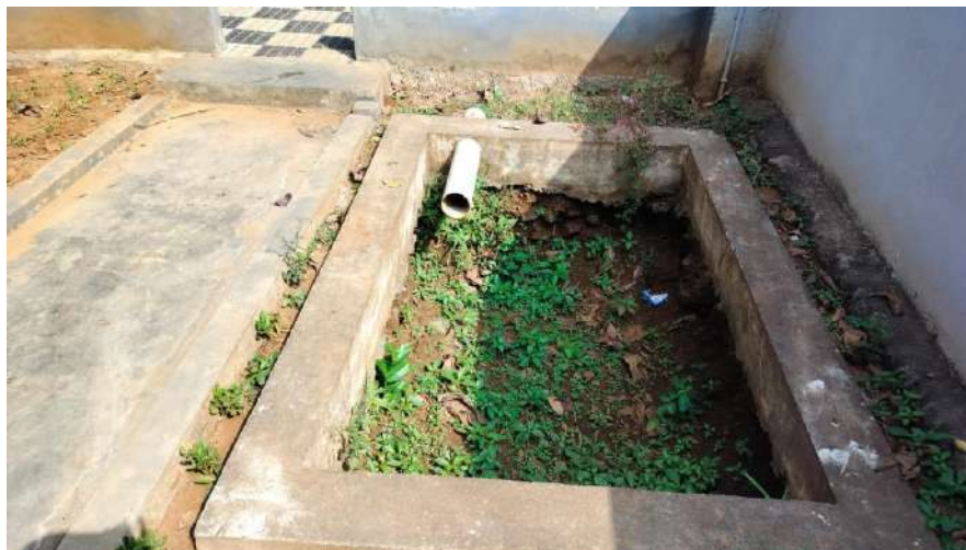
RAIN WATER STORAGE TANK – 2 IN VOCATIONAL COURSES BLOCK
